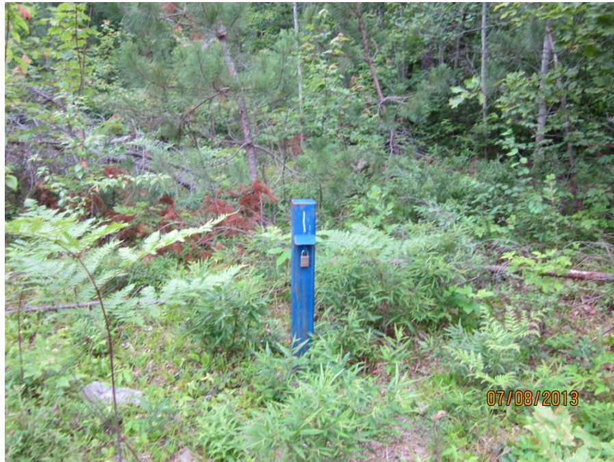
Photo 5 Groundwater monitoring wells BH4, July 2013
