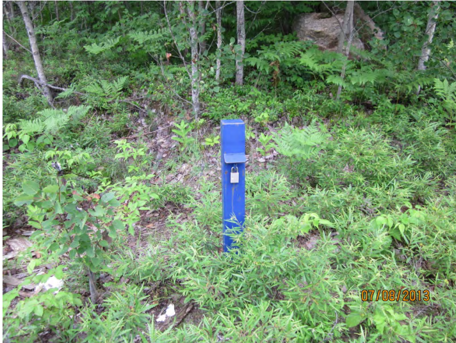
Photo 7 Groundwater monitoring wells BH6, July 2013
