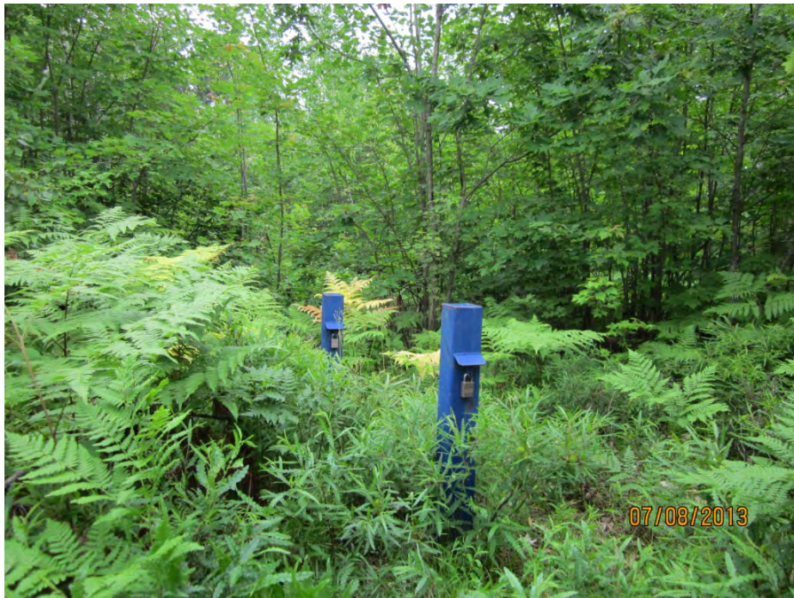
Photo 4 Groundwater monitoring wells BH3-I and BH3-II, July 2013
